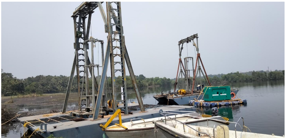
Figure: Floating solar project marine construction platform and equipment
