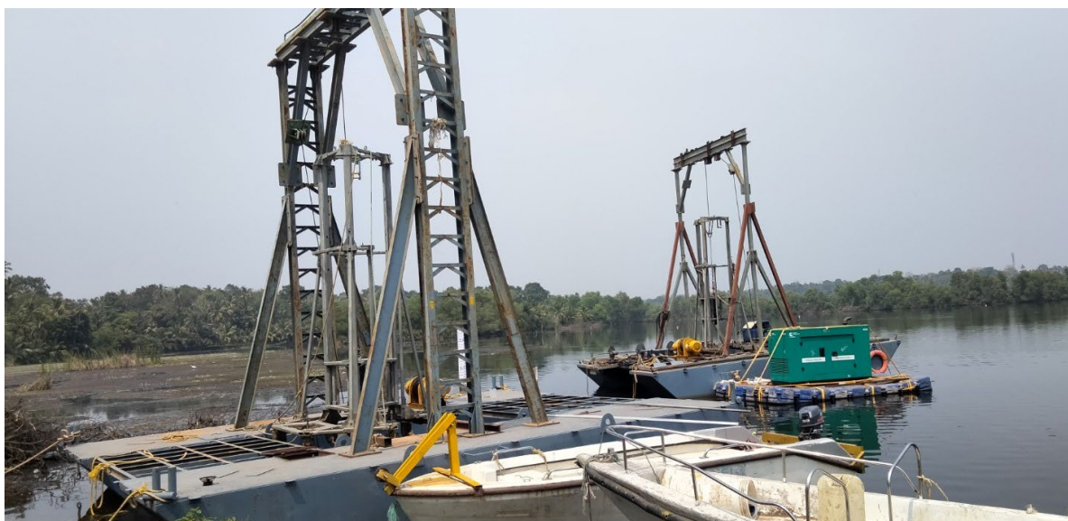
Figure: Floating solar project marine construction platform and equipment
